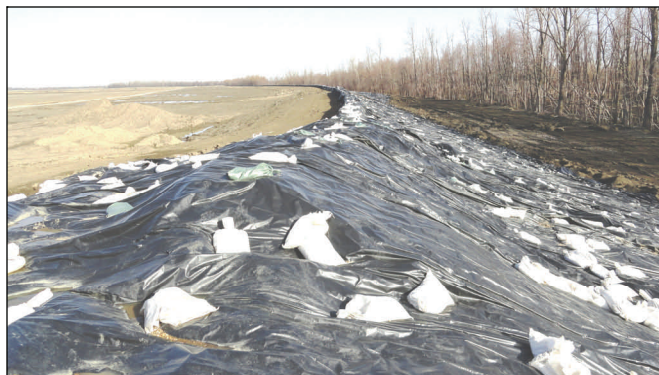
Plastic sheeting to protect the levee and HESCO barriers is shown in this March 1 view.
